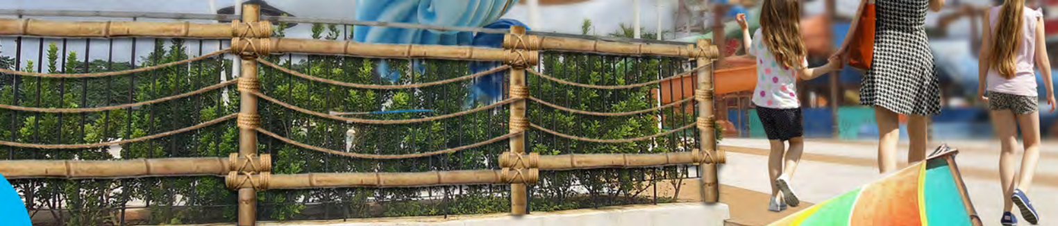
BAMBOO RAILING ACCENTS: Bamboo FRP cladding with manila rope assembly.
