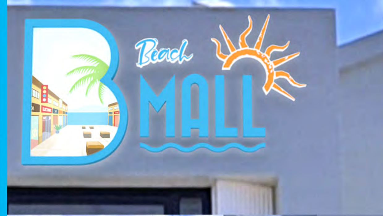
Build up Letters and Wave with UV sticker (for color) with backlight and acrylic cover at
